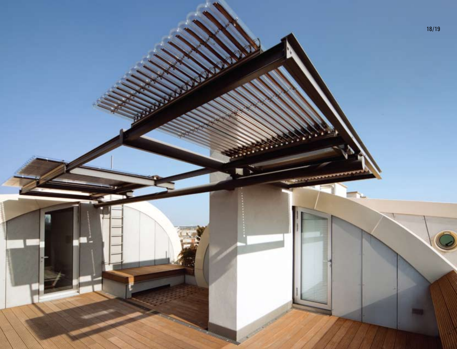
Example of using Vitosol 200-T tube collectors.
